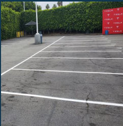
Parking lot striping
