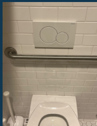
Specialty part installation
